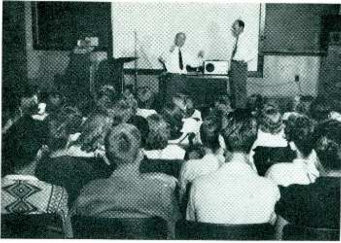
The drill room is the simplest form of electronic teaching. Here a tape recorder is used to play a master tape to an entire class which then repeats in unison. By the addition of jack boxes, shown at right, the unit may be converted into a listening post. The students wear headphones and achieve some degree of isolation. Such a listening post can be set up in a school library or other spot.
